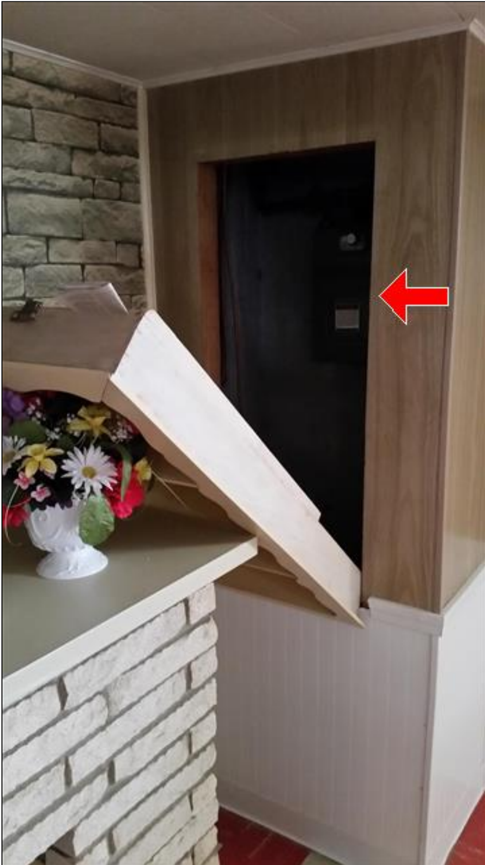
5.1 Item 1(Picture) Natural gas shut-off is located behind a "hidden-panel"
