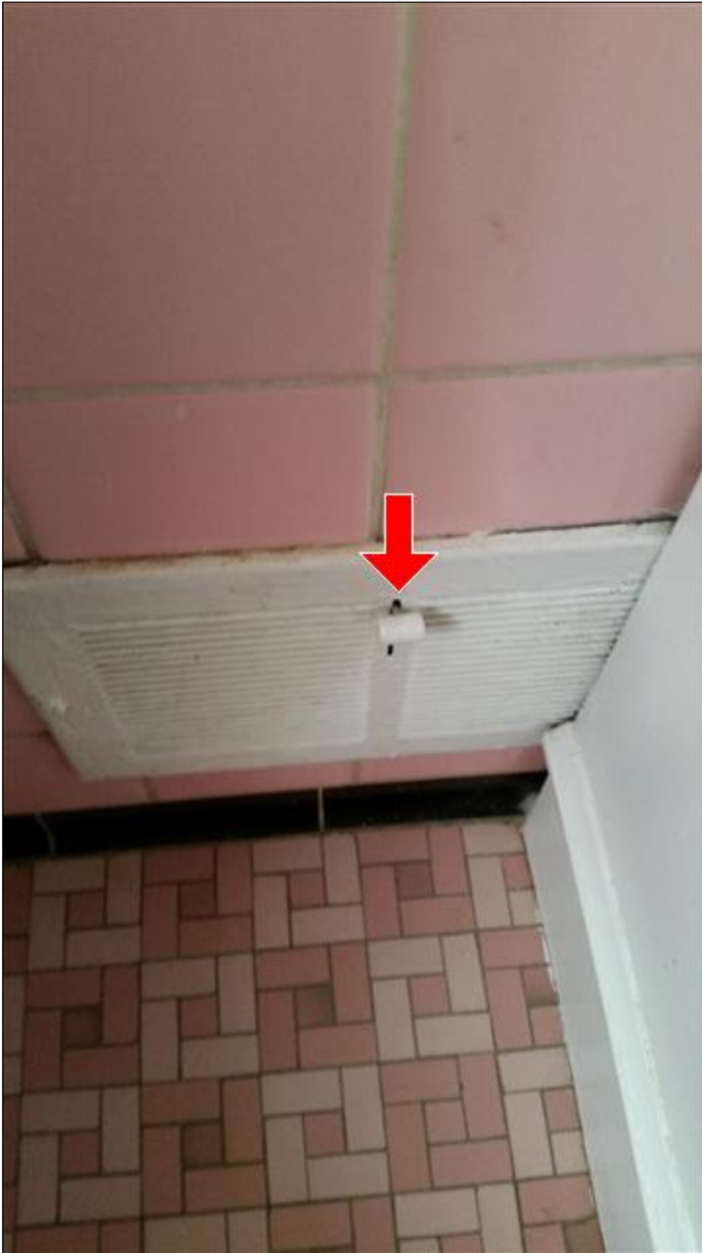
4.3 Item 1(Picture) Vent cover with adjustable damper lever is difficult to move
